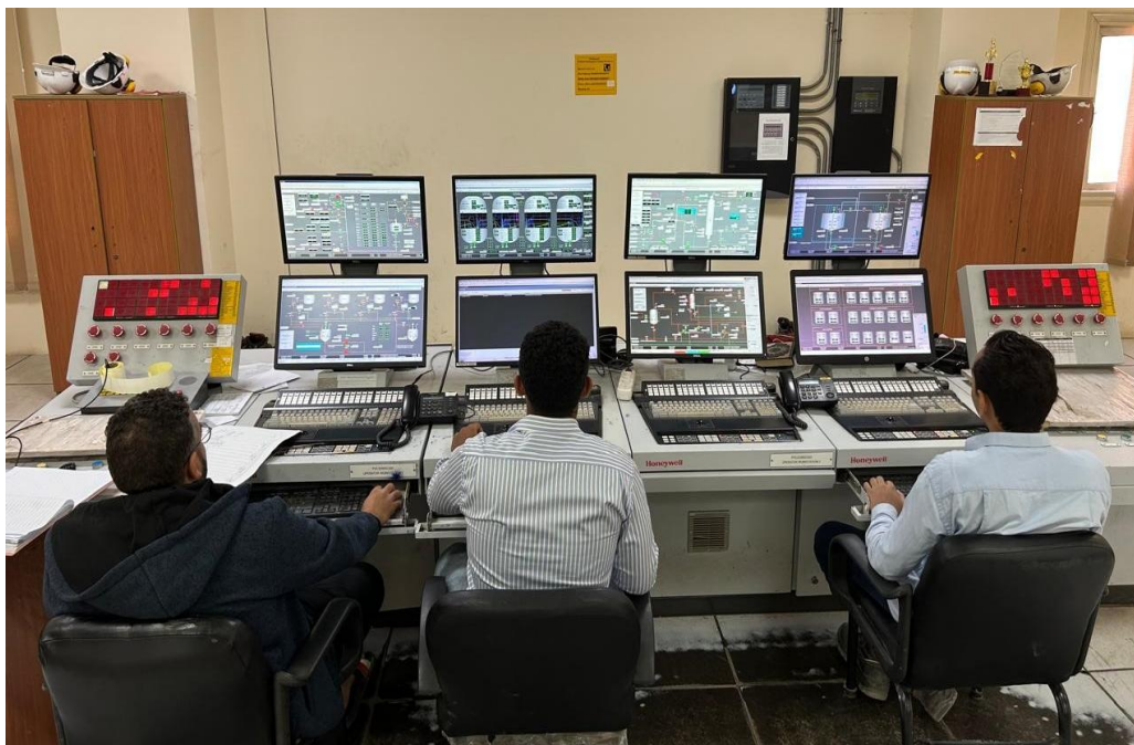
PVC Plant Process control and DCS Training
